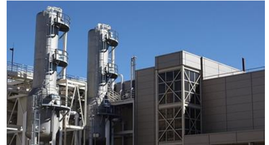
West side of Central Utility Building (CUB) with view of gas towers and ultrapure water (UPW) tanks.
