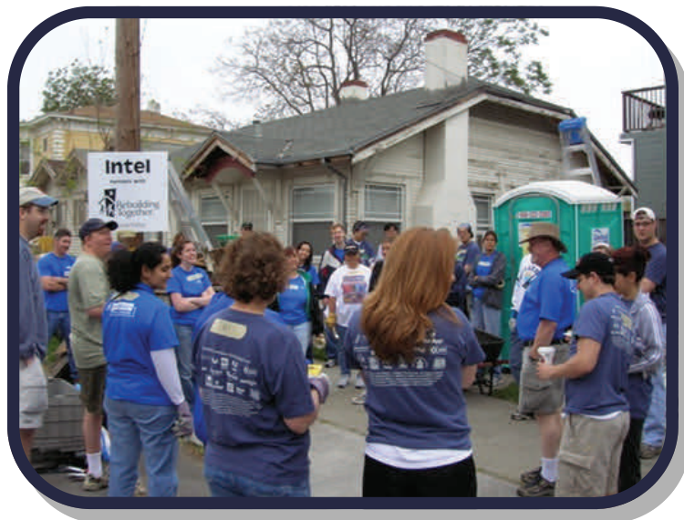
Lonnie as "House Captain" on a Building Together site involving almost 40 Intel employees over three weekends
